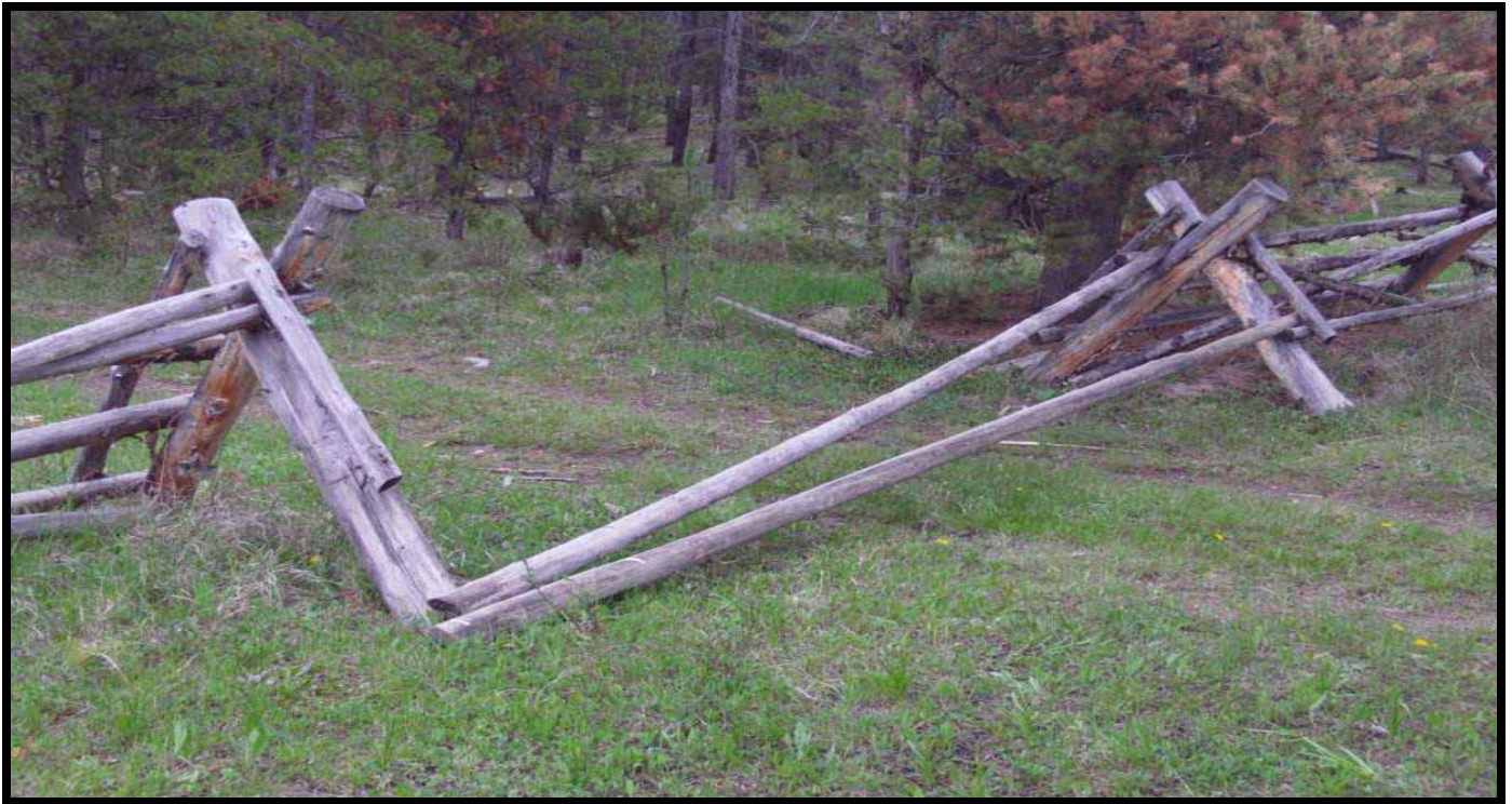
Recommended wildlife-friendly dropped rail crossing structure on a fence in the Big Hole watershed. Photo: Hans Humbert
