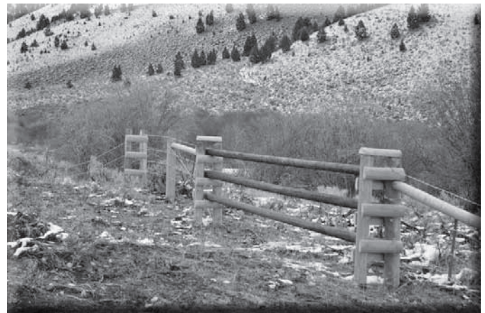
Wildlife crossings allow elk and moose to easily cross the fence without damaging it.
