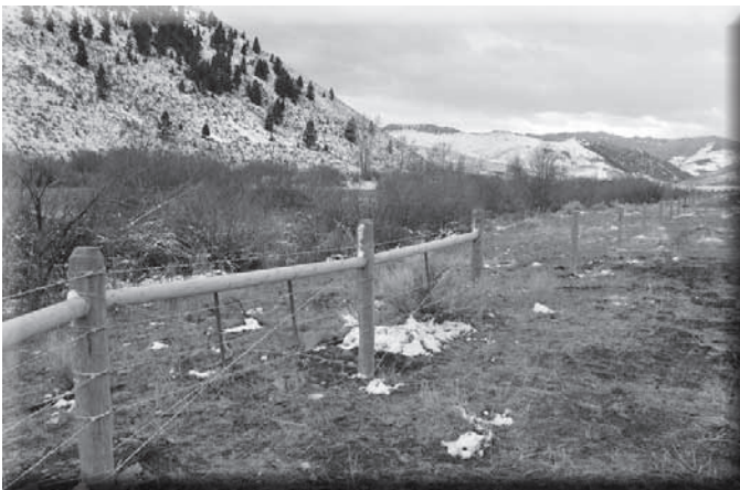
Newly installed fence ties into existing permanent fences.
